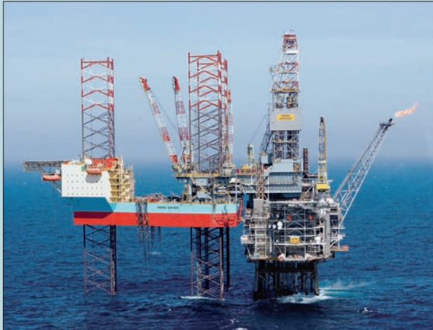
The drilling rig "Maersk Inspirer"
