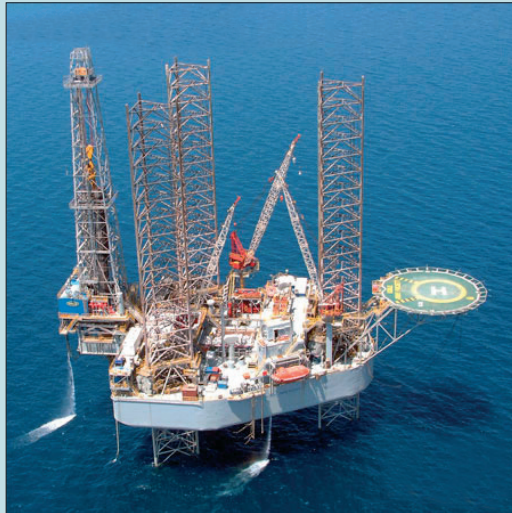
The drilling rig, "Jimmy Puckett", Noble Corporation
